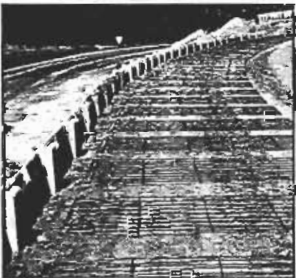
Mechanically Stabilized Embankment, bar mats in position.
