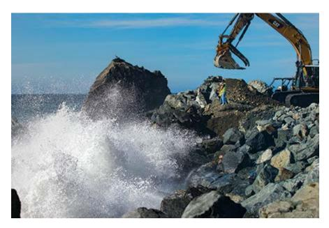
From fall 2017 to winter 2018, several large storms in the northern Pacific Ocean caused large swells and breaking waves at the project site, hampering construction of the rock revetment at the toe of the slide. KYLE EVANS 2018
