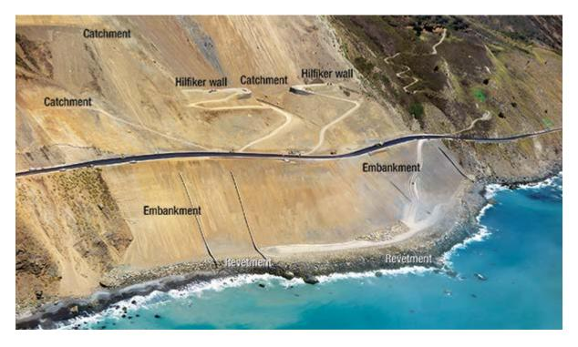
The main features of the completed project included a rock revetment at the toe of the landslide to control erosion, a new embankment built up from the revetment, and large earthen berms outfitted with a type of rock basket wall known as a Hilfiker wall to capture materials that travel downslope from the catchment above. COURTESY OF JOHN MADONNA CONSTRUCTION
