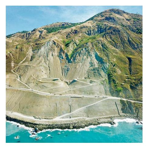
To reopen State Route 1 as quickly and as safely as possible, Caltrans opted to construct a newly relocated highway across the body of the landslide. COURTESY OF JOHN MADONNA CONSTRUCTION
