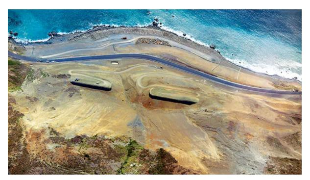
At the Mud Creek site, the rock basket walls were built up to about 25 ft in face height, dramatically improving the ability of the above-roadway catchments to protect the new highway below. COURTESY OF JOHN MADONNA CONSTRUCTION
